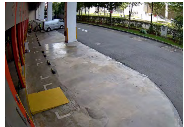
> Sample FOVs from newly installed overlooking various operation functions (Project NorthStar)
